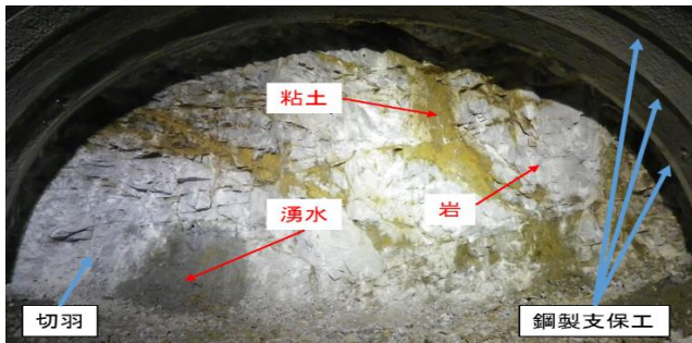
Fig.1 Tunnel face image
