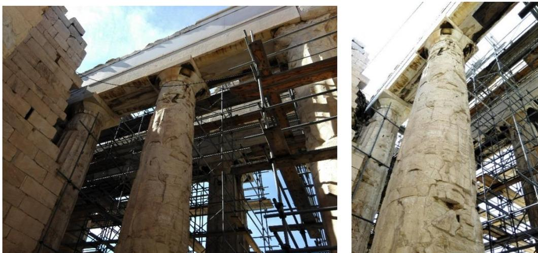
Fig.1-5: Internal column damaged by historical fires on the west side
