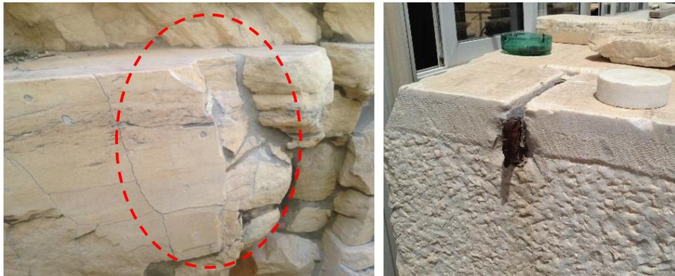
Fig.1-8: Former restoration using normal concrete and iron clamp
