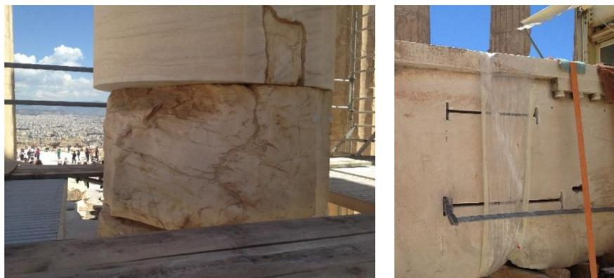
Fig.1-9: Present restoration using white cement and titanium clamp
