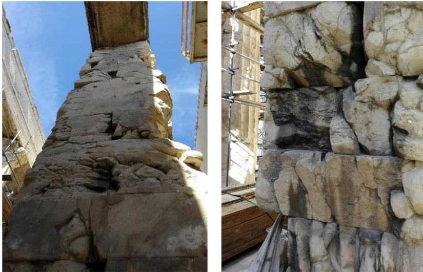
Fig.1-6: Wall damaged by historical fires on the west side
