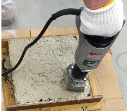
Photo 3.3 Mortar filling technique
