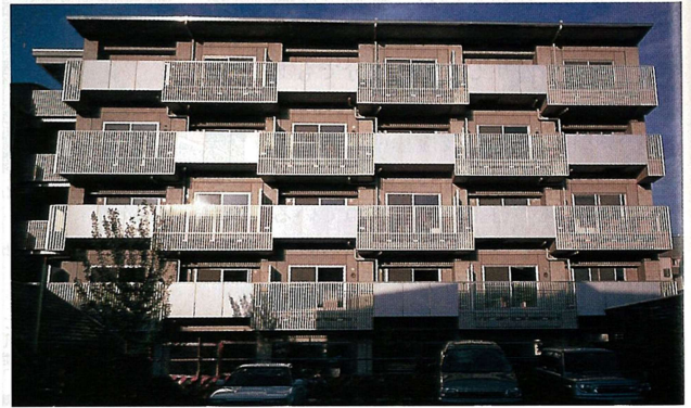
Characteristic facade emphasizing "checkerboard" slab system
