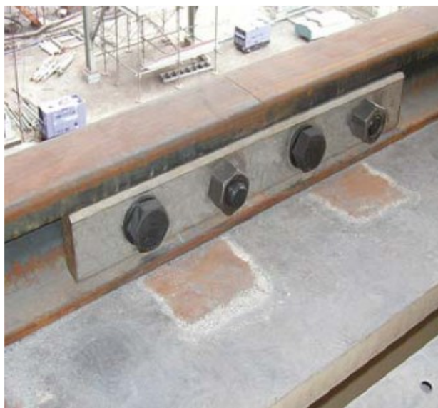
Fig.2-2 Locking joint of Fe-Mn-Si-Cr shape memory alloy (23) .
