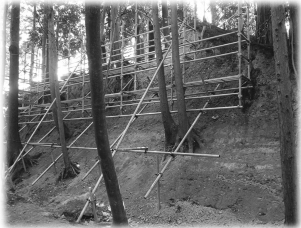
Figure 9: Remains of wall, Kannon Mountain section. Photos by author.
