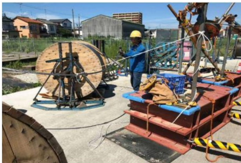
Fig.2.4 Winch operation on the ground
