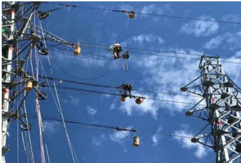
Fig.2.5 Electric wire embarking in the air
