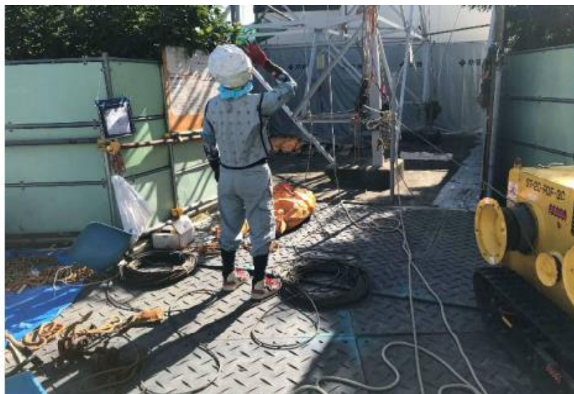
Fig.2.1 Ground work on iron plate
