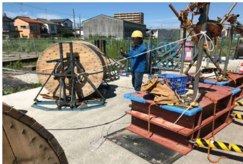
Fig.2.2 Winch operation on the ground
