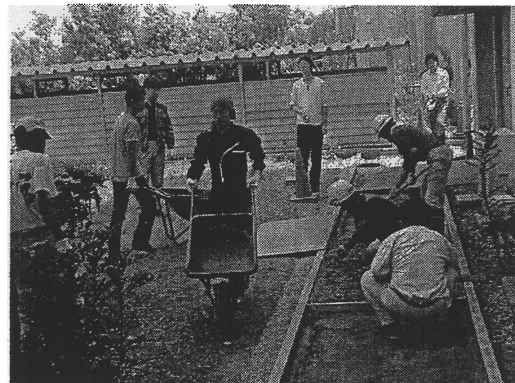
Figure 2.35 Placing in progress
