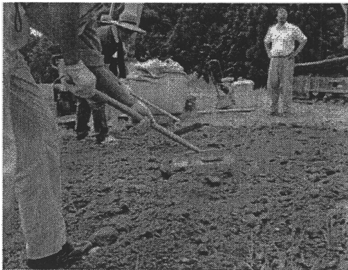
Figure 2.13 Leveling of the site with the hand
