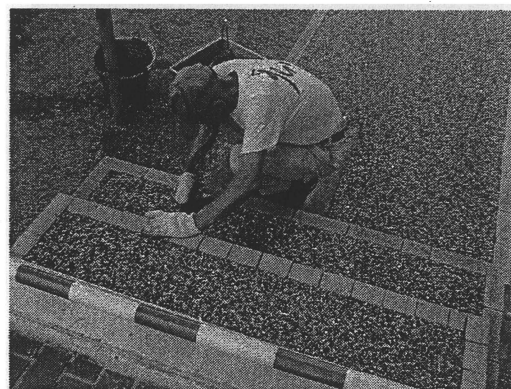
Figure 2.44 The upper layer is about 1 cm
