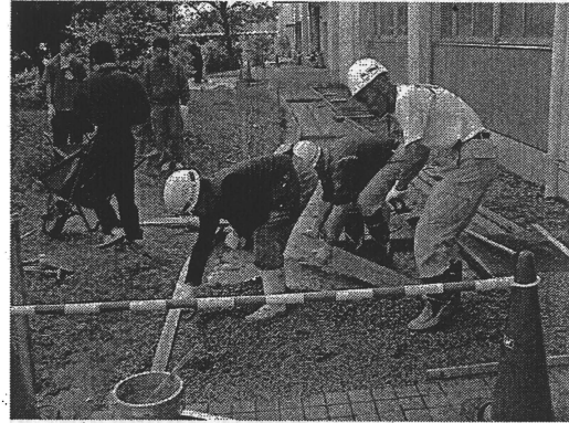
Figure 2.33 Placing and laying of POC
