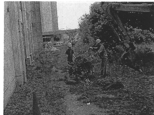
Figure 2.10 Clearing of the site for placing of T.N. Base pavement
