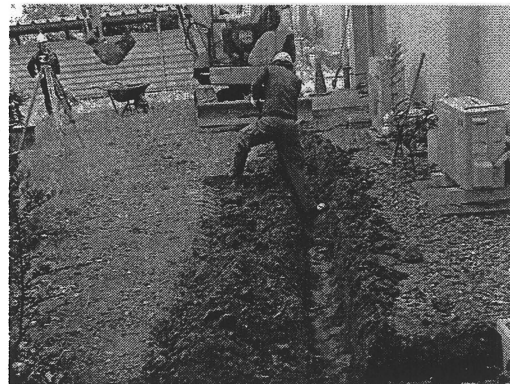
Figure 2.16 Drain for placing of drainage pipes
