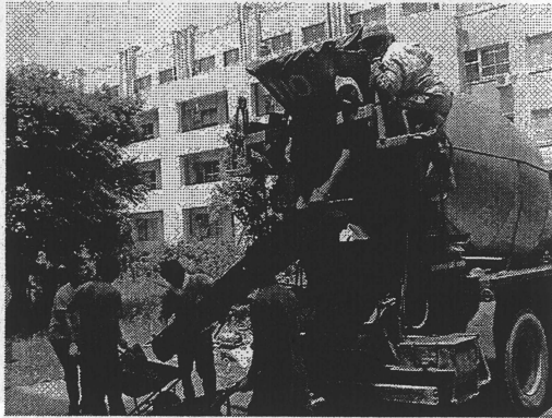
Figure 2.30 Fresh concrete from a concrete mixing plant
