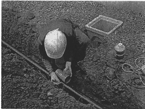
Figure 2.18 Laying of pipes for the drainage
