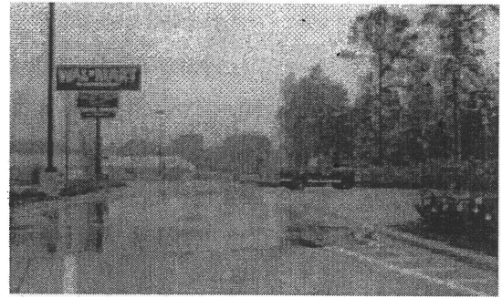
Figure 2.3 POC and asphalt pavements after a rainfall [10]
