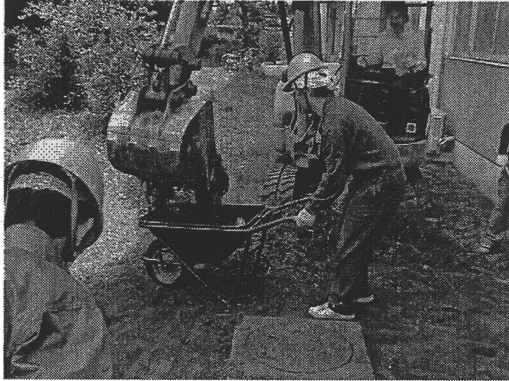
Figure 2.12 Clearing the debris from the site
