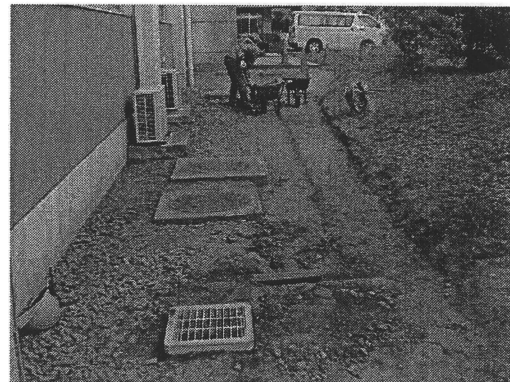
Figure 2.22 Leveling back after drainage pipes have been laid
