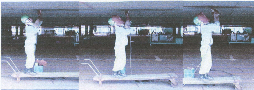
(a)Gauging (b)Welding (c)Grinding
