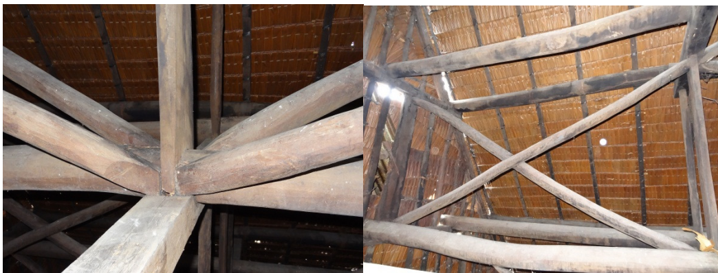
Photo.3-18 Detail of braces at roof structure
