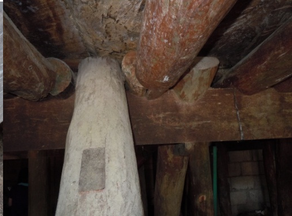
Photo.3-12 Brace for ridge direction
