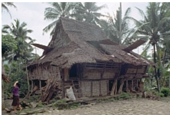
Photo.1-3 Traditional house in Central Nias (source: Sato.K)
