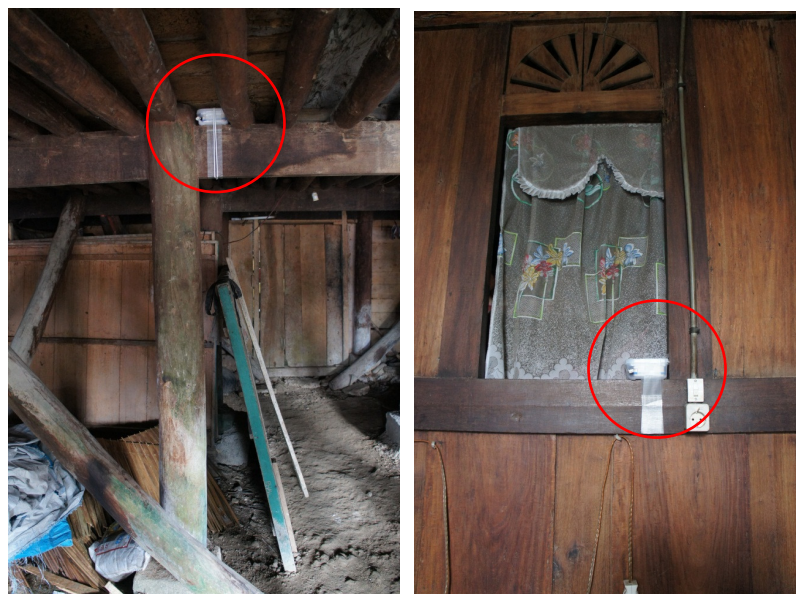
Photo.4-4 Arrangement of the sensors (left: understructure, right: living space)
