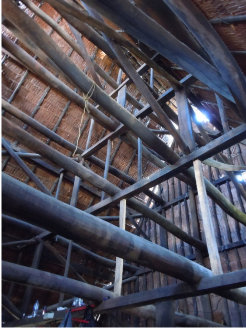
Photo.3-19 Inside roof frame
