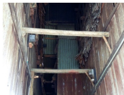
Photo.3-7 Above the passage
