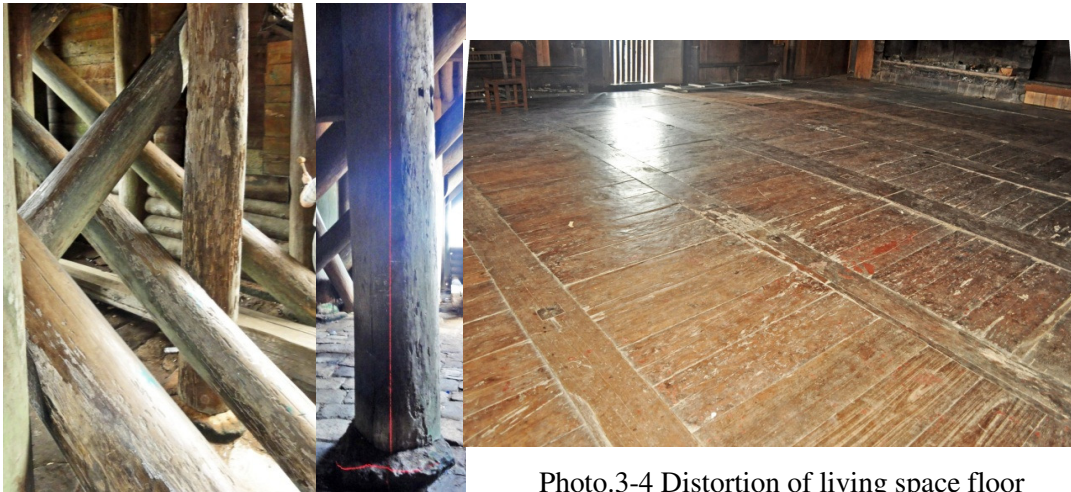
Photo.3-3 Bite mark of termite and laser light of Laser Marking Equipment
