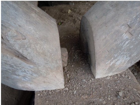
Photo.3-11 Base of front brace
