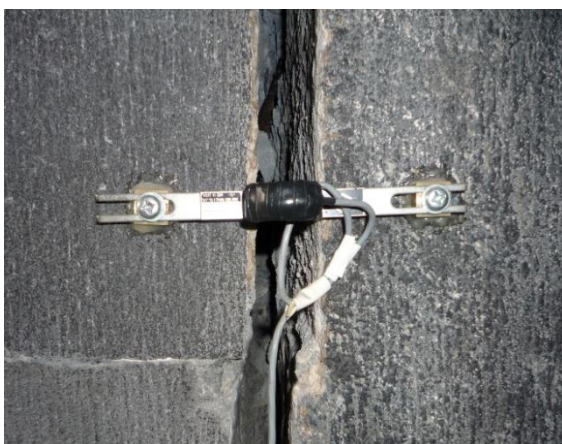
Fig. 3-114 View of displacement transducer (PI-2-100)
