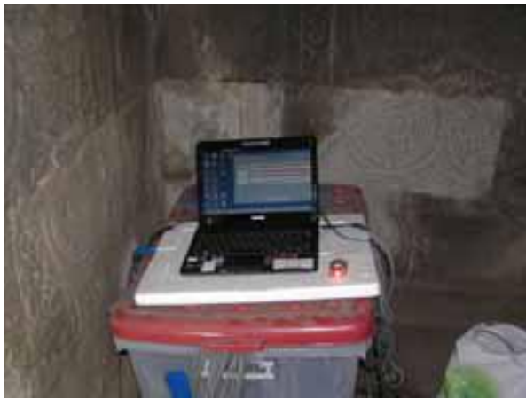
Fig. 3-13 View of NTP Server
