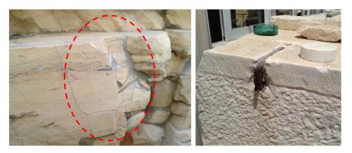
Fig.1-8: Former restoration using normal concrete and iron clamp
