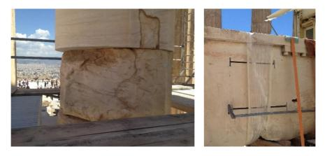
Fig.1-9: Present restoration using white cement and titanium clamp
