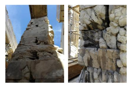
Fig.1-6: Wall damaged by historical fires on the west side
