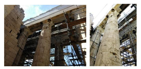
Fig.1-5: Internal column damaged by historical fires on the west side
