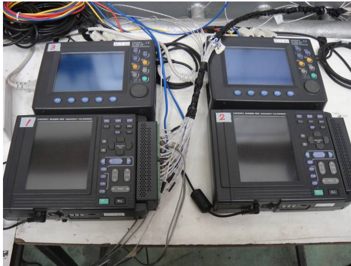
Fig. 4-4 Data loggers and power meters set up
