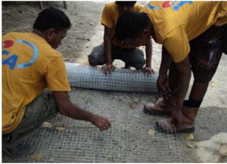
(A) Setting wire mesh (cutting and bending): It is better to bend before assembling for corner and top of walls.
