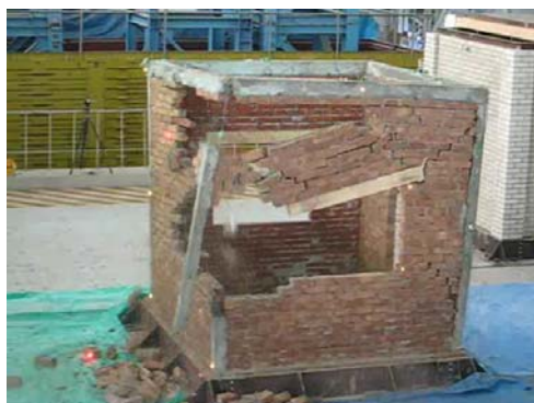
5. Separated RC column from RC beam.
