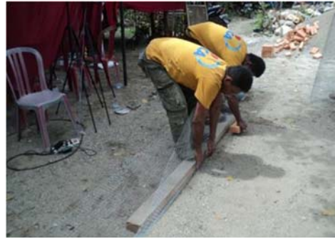
(A) Setting wire mesh (cutting and bending): It is better to bend before assembling for corner and top of walls.
