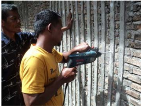
(B) Making through holes for fixing wire is made by drilling, diameter 10 mm on the joint mortar.
