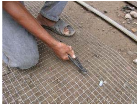
(A) Wire mesh: Galvanized Welded Wire mesh, Spacing 25 mm, 1 mm Diameter
