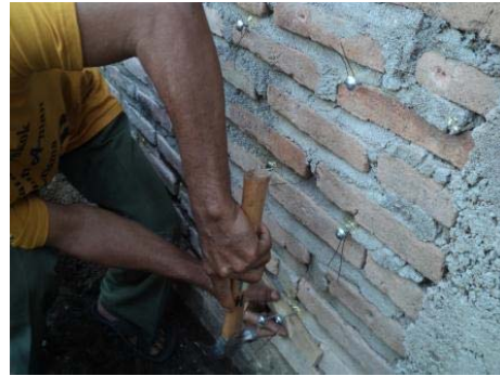
(B) Making through holes for fixing wire is made by drilling, diameter 10 mm on the joint mortar.
