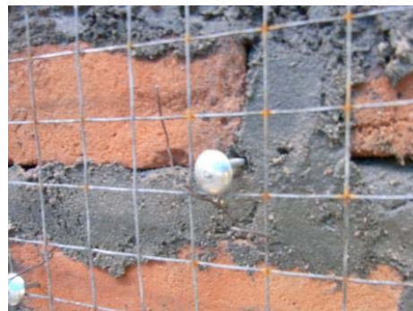
(D) Inside and outside wire mesh is stitched, using tie wire inserted through holes in the wall.
