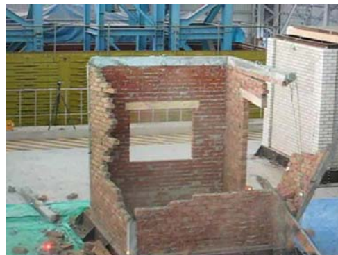
8. Falling down of East wall
