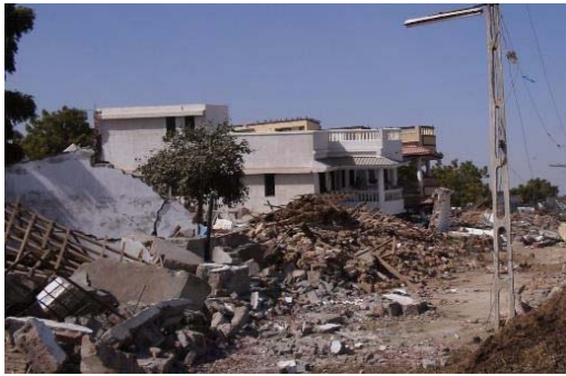
(A) 2001 Bhuj earthquake in India, adobe and brick masonry were damaged
