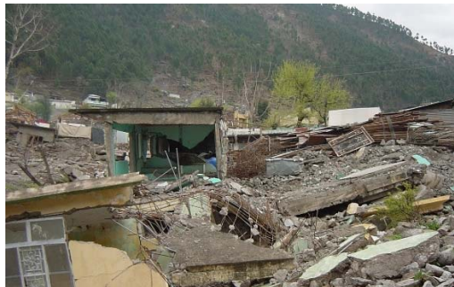
(C) 2005 Kashmir earthquake in Pakistan, stone and CB masonry were damaged
