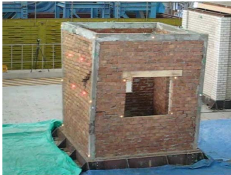
1. First, collapse of walls occurred in the West wall.
