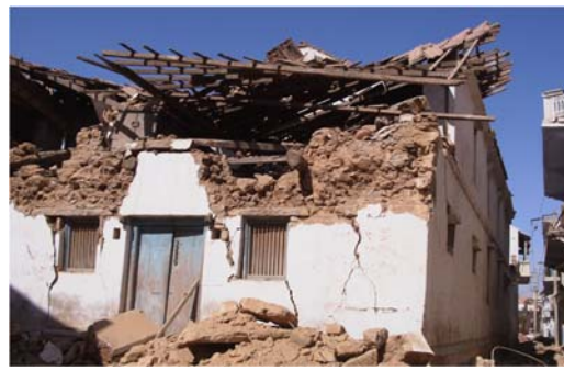
(A) 2001 Bhuj earthquake in India, adobe and brick masonry were damaged
