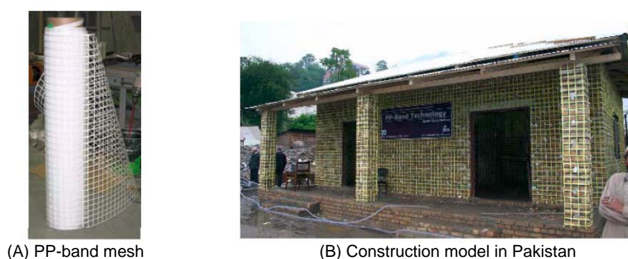
Fig.17 PP-band mesh retrofitting by K.Meguro
