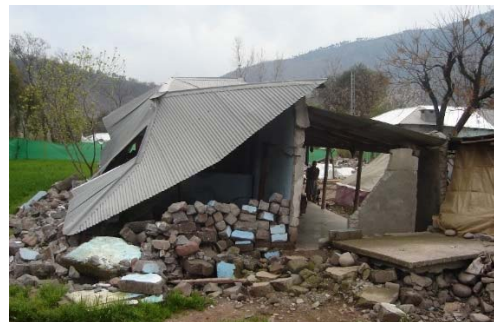
(C) 2005 Kashmir earthquake in Pakistan, stone and CB masonry were damaged
