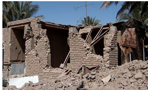
(B) 2003 Bam earthquake in Iran, adobe and brick masonry were damaged
