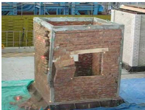
3. Collapse of the South wall started.
