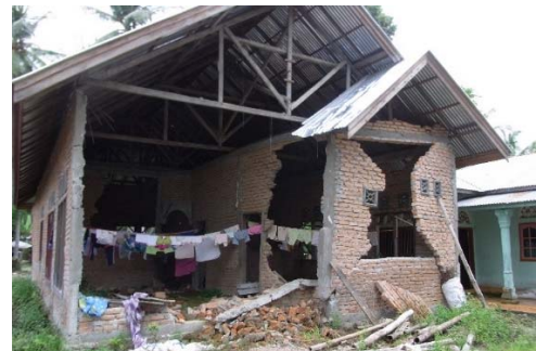
(D) 2006 Central Java earthquake, 2008 Sumatra earthquake (Padang) in Indonesia, brick masonry and confined masonry were damaged
