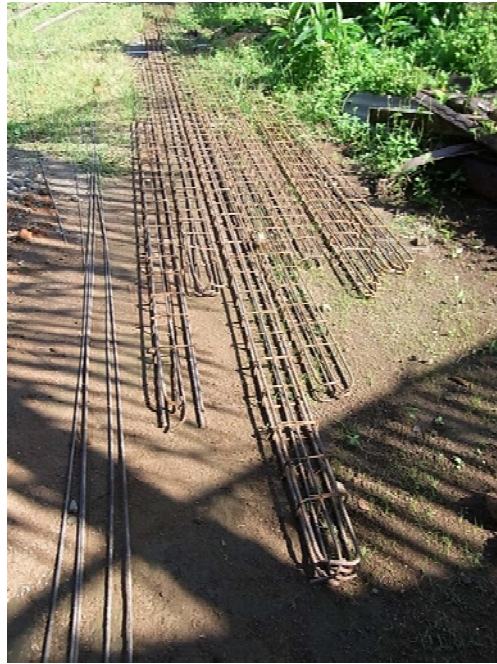
Fig.146 Assembled reinforcement units
