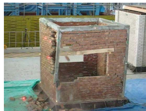
4. The part of the South wall, side of opening fell down.
