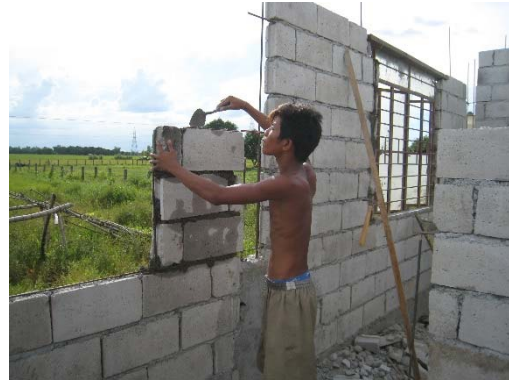
Fig.25 Non-engineered construction in Philippines
