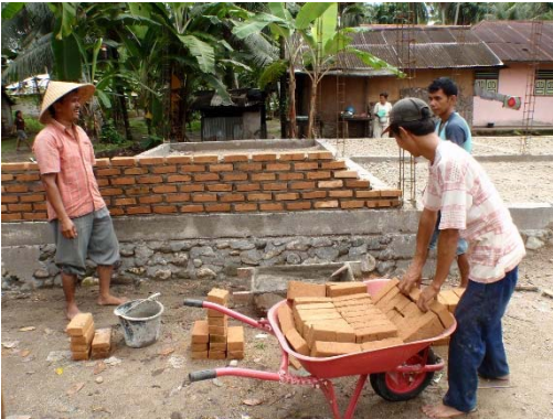
Fig.24 Non-engineered construction in Indonesia
