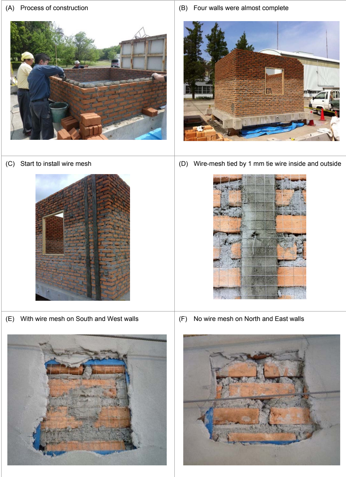
Fig.100 Process of construction of Model
