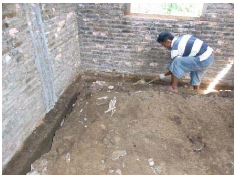
(E) Wire mesh should be installed from bottom to top.
