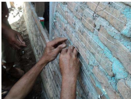
(D) Inside and outside wire mesh is stitched, using tie wire inserted through holes in the wall.
