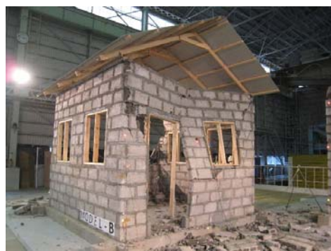
Fig. 86 Out-of-plane failure in shaking table test of CHB model structure in Chapter 2.4
