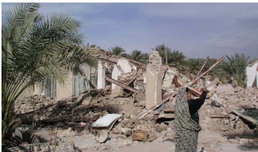
(B) 2003 Bam earthquake in Iran, adobe and brick masonry were damaged
