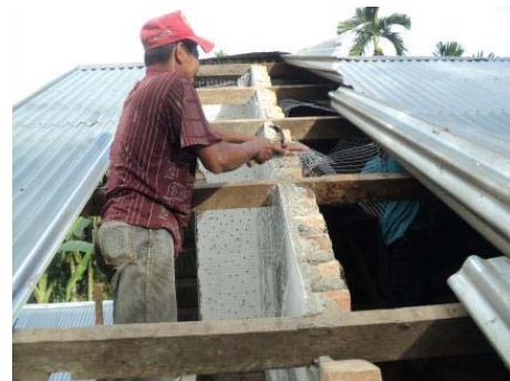
(D) Inside and outside wire mesh is stitched, using tie wire inserted through holes in the wall.
