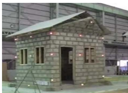
Fig. 90 Out-of-plane failure of gable wall in shaking table test of CHB model structure in Chapter 2.3
