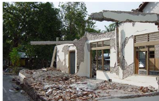
(D) 2006 Central Java earthquake, 2008 Sumatra earthquake (Padang) in Indonesia, brick masonry and confined masonry were damaged
